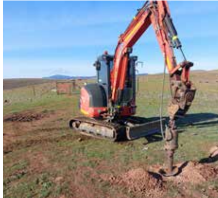
Excavator in action digging holes.
