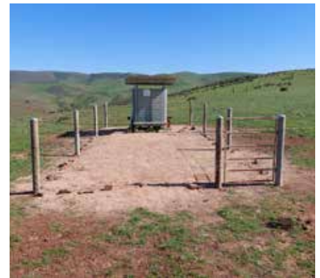
End of the first day of work.
